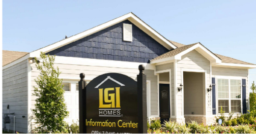
Project Progress: Park Vista at El Tesoro 6498 Selinsky, 77098 (District D)
