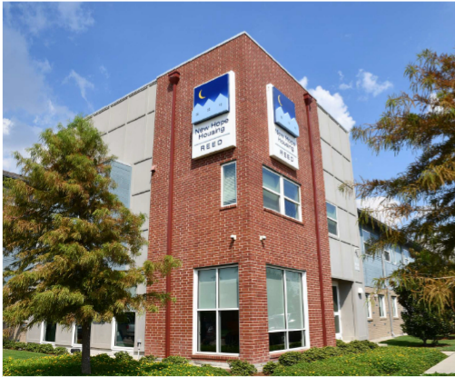
Project Progress: NHH at Reed Road 2605 Reed Rd. 77051 (District D)
