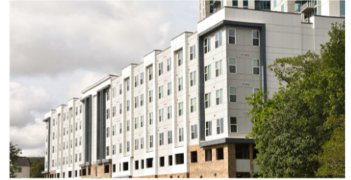
Update: Gala at MacGregor New Construction 102-120 Carson St., Houston, 77004 (District D)
